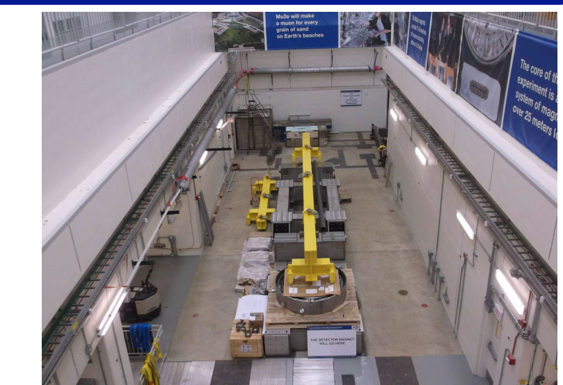
Mu2e experimental site in construction @ Fermilab
