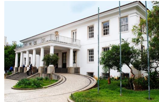
Rectory - located at a Historical Building
