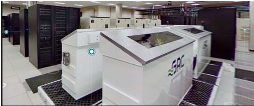
Liquid-Immersion Cooled (Frontera - TACC)
